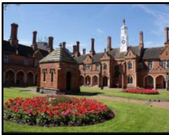
The Almshouses After
